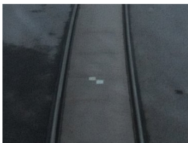
Signal marker painting on a tram track
